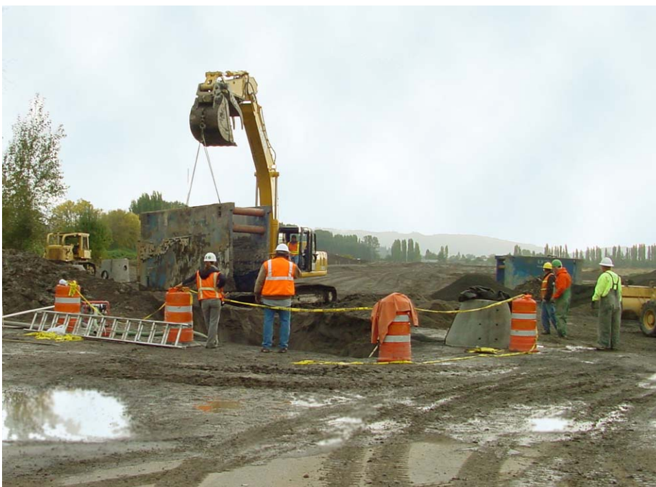
Crocker Avenue Extension Project at the Mint Farm Industrial Park.
