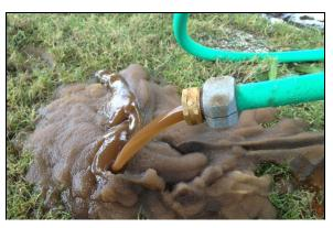
Sediment Removed during Ice Pigging
