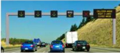
Figure 10: Lane Control and Supplemental Signs on Gantry
