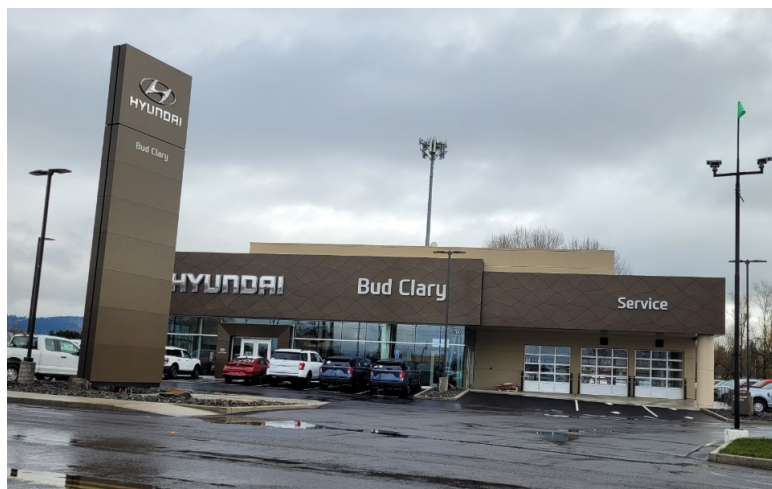
BUD CLARY HYUNDAI BUILDING UPDATES AND SHOWROOM RENOVATION NEARING COMPLETION.
